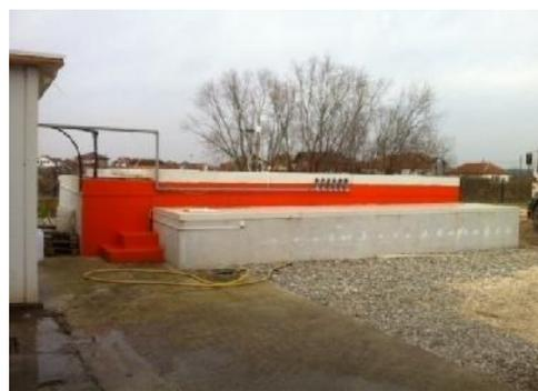
**Figure 2:** Sequencing batch reactor in the dairy industry
