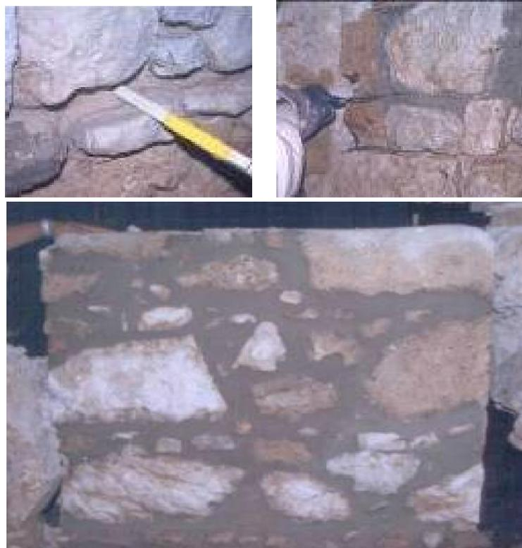
**Figure 1.** Grout injection procedure, drilling holes in mortar joints and fixing
