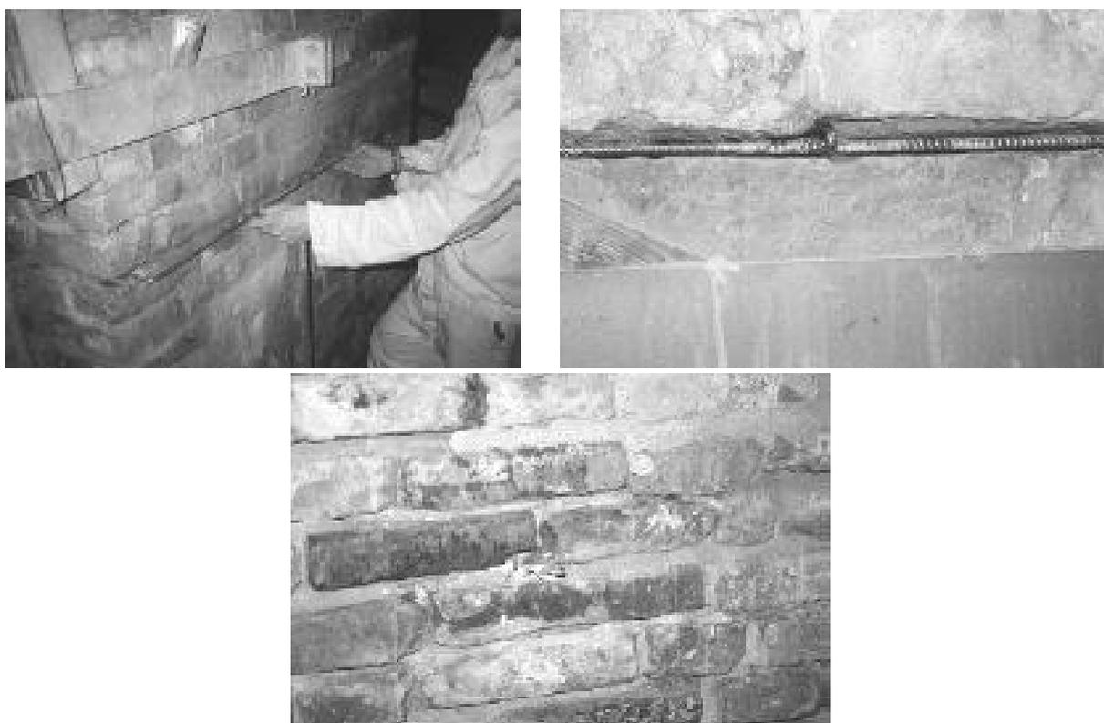
**Figure 7.** Execution stages in the case of reinforced re-pointing performed
