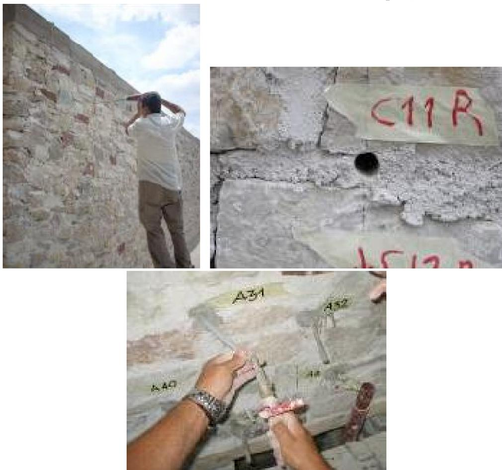
**Figure 5.** Grout injection procedure, drilling holes in mortar joints and fixing
