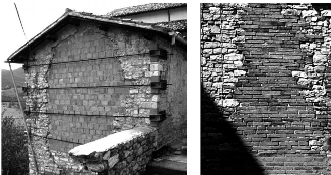
**Figure 9.** Masonry replacement intervention
