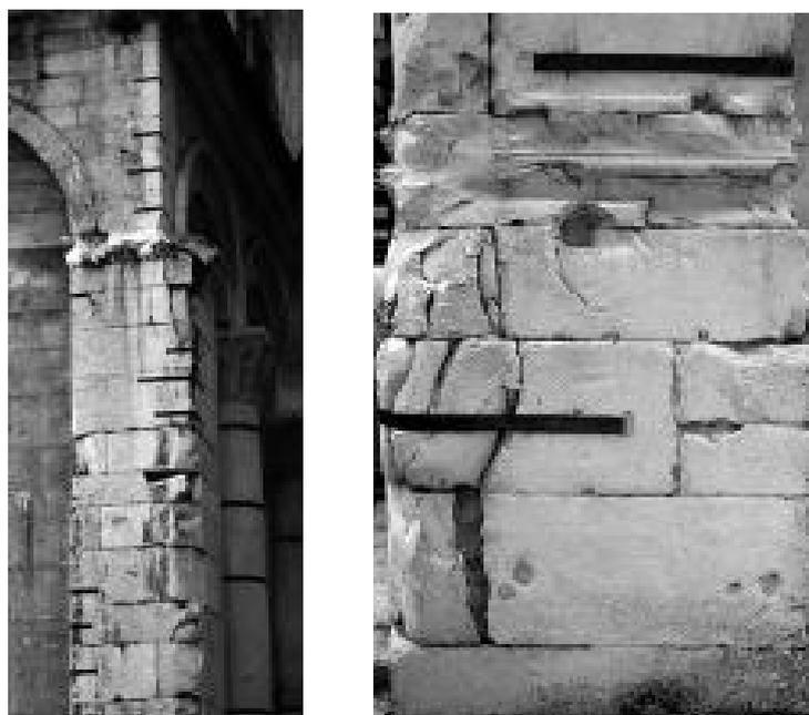
**Figure 2.** Crack fastening by metal bars
