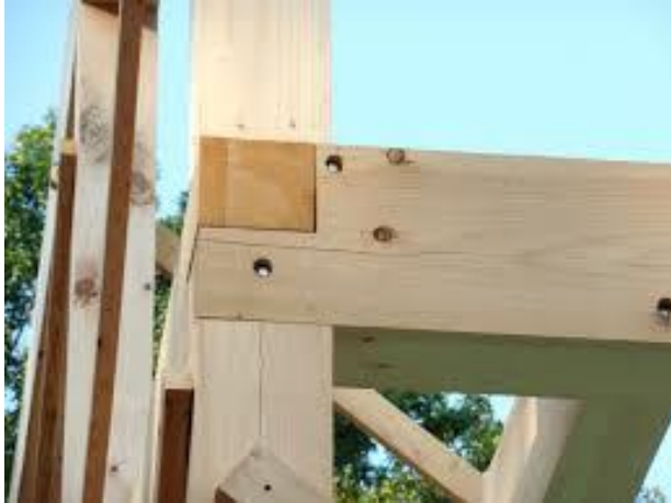
Figure 1. An example of mechanical fasteners used in wooden constructions
