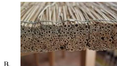
**Figure 1.** Reed bladed slabs from longitudinally located sheaves (stems thickness 0.2 - 0.5 cm).
